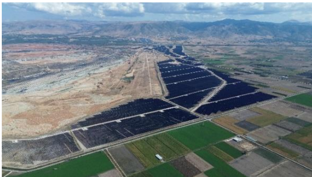
Figure 1: Part of a 550 MW photovoltaic facility located near the Agios Dimitrios Power Plant.
