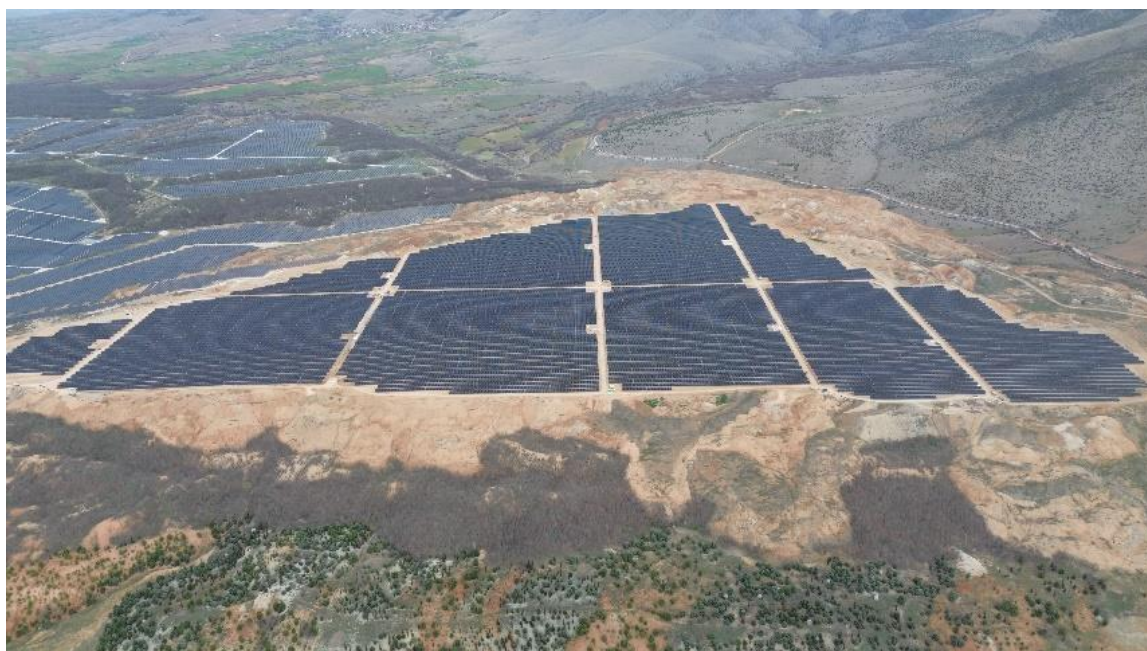
Figure 2: Section of a 171 MW photovoltaic plant located in a former deposition area of the Western Macedonia Lignite Center.
